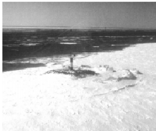
b. Closeup of the ice island. It is constructed of quarried rock, the top diameter being roughly 40 feet.
