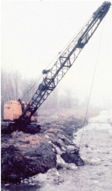
Figure 3-10. Using a bucket dredge to break ice in a river.
