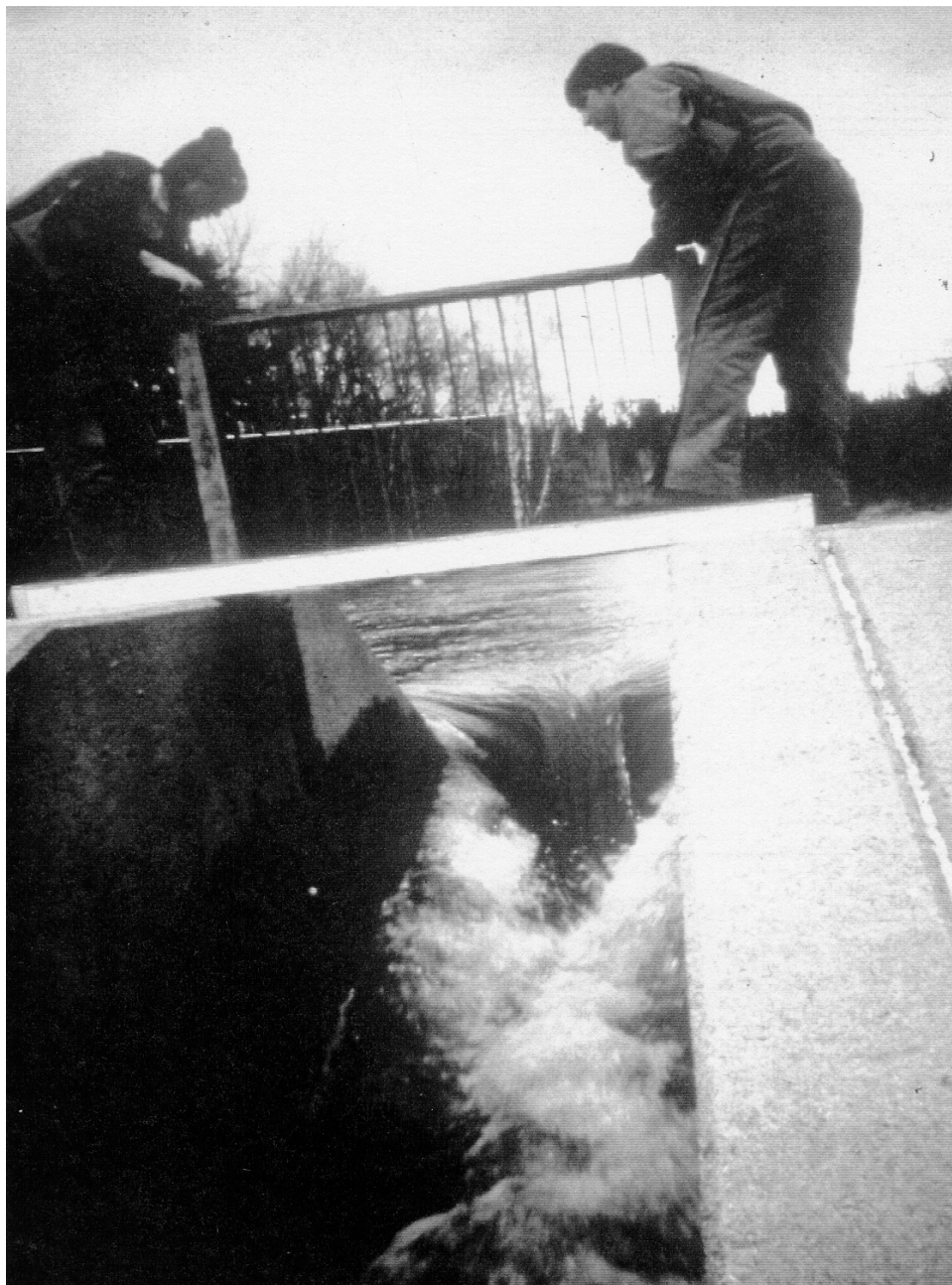
a. Installing racks in sluiceways
