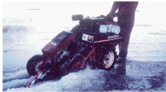
b. Ditchwitch 1260 cutting ice in Montpelier, Vermont.
