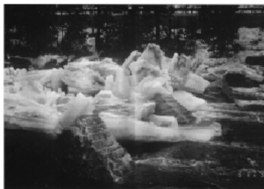
Figure 3-34. Cut granite block ice control structure in Hardwick, Vermont, following breakup, March 1995.
