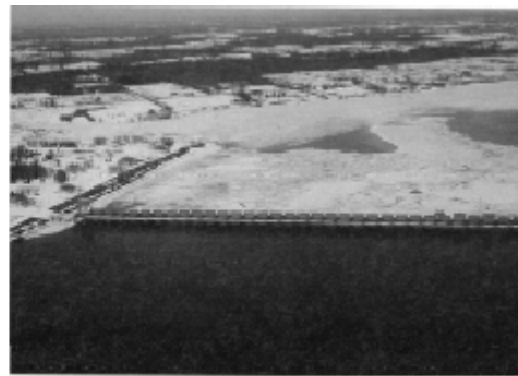
c. Iroquois control structure.
