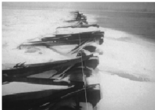
Figure 3-22. Boom on Beauharnois Canal, constructed of double steel pontoons.
