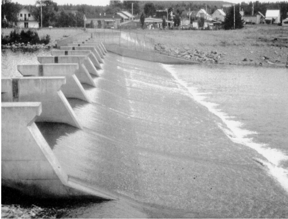
Figure 12-5. Ice piers for breakup control
