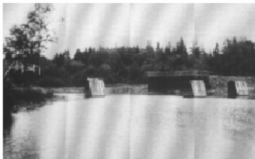
Figure 3-36. Rock-filled timber cribs upstream of the dam at Cherryfield, Maine.
