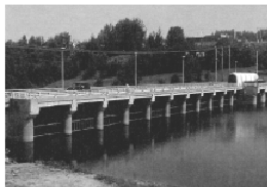
b. Upstream side, showing the ice retention grates.
