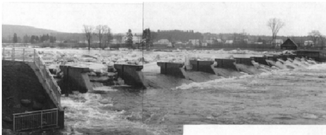
Figure 3-35. Weir with piers ice control structure on the Ste. Anne River, St. Raymond, Quebec. (Photo courtesy of Marc Delagrave, Roch Itée Groupe-conseil, Sainte-Foy, Quebec.)
