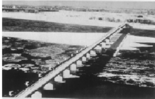
Figure 18-4. Montreal Harbor ice control structure. (From Lawrie 1972.)
