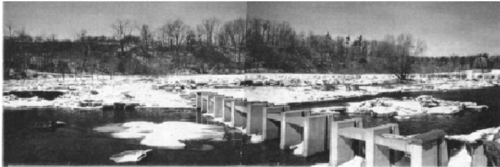
Figure 3-33. Credit River ice control structure following breakup, March 1994. Note the ice stored on the right flood plain. (Photos courtesy of Harold Belore.)
