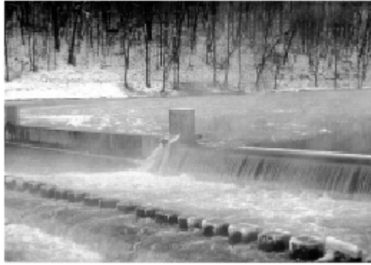
Figure 3-28. Ice control weir on Oil Creek, upstream of Oil City, Pennsylvania.
