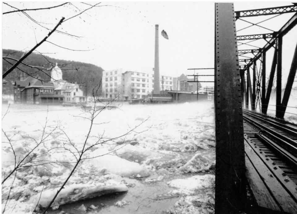
Figure 1-5. Flooding caused by an ice jam
