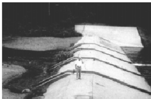
Figure 3-27. Ice control weir on the Israel River, Lancaster, New Hampshire, July 1994.
